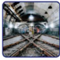
Metro/Train Road Tunnels
